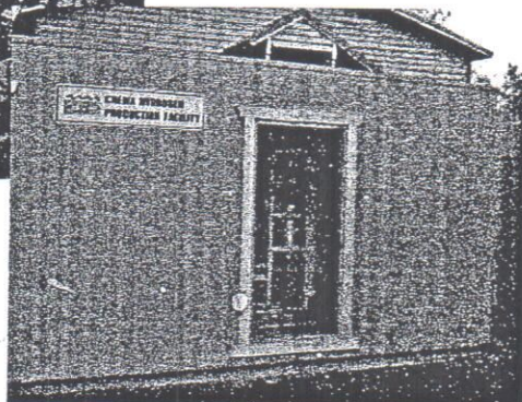
Hydrogen Production Facility at Chena
